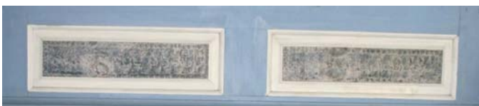
Example of the Mantel Detail in the Mansion, 2007
