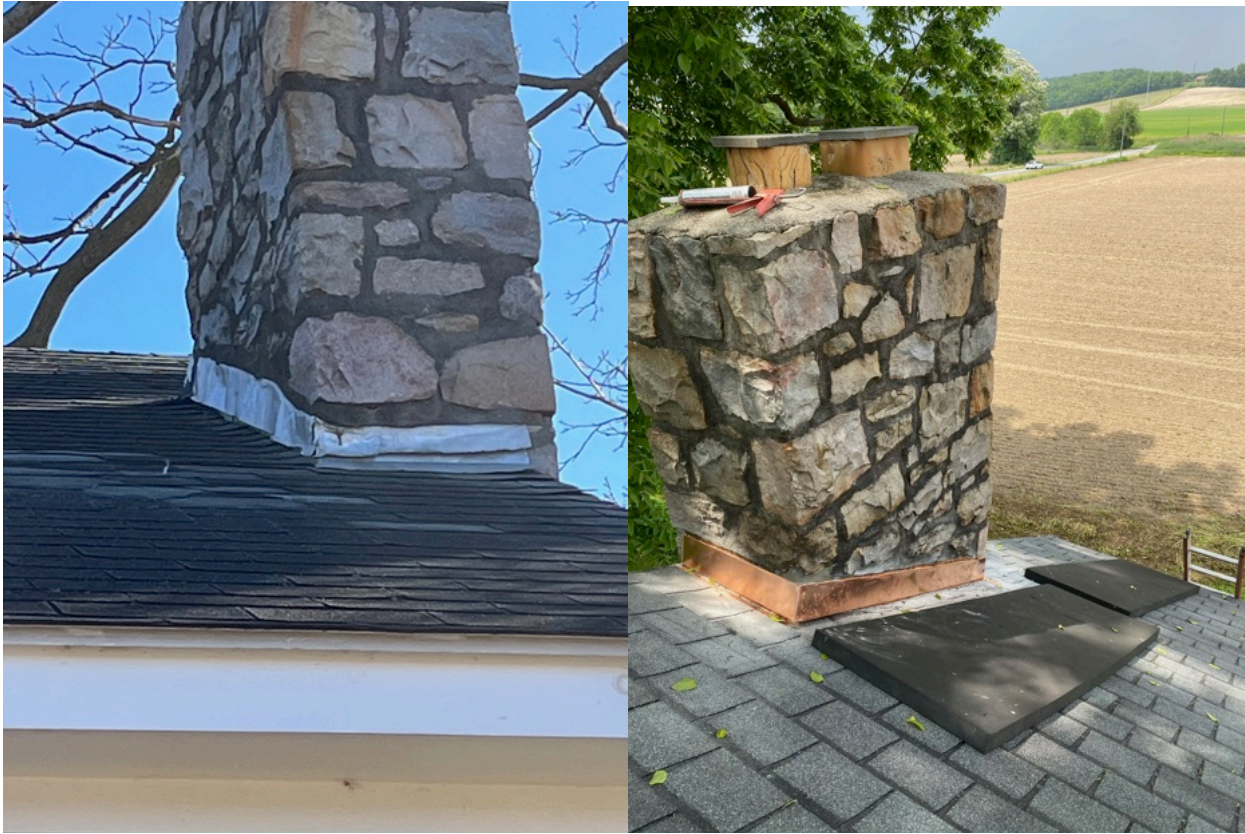
Rear slope partially roofed, chimney flashing before and after.
